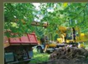
Work on the soil layer recovery
